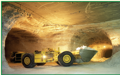
Mining operation to recover kieserite
