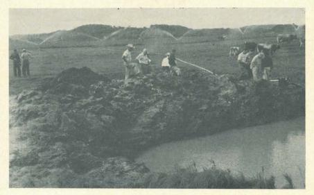
From this water hole, a 7-horse motor and pump delivered water to 16 sprinklers spraying the 6-acre demonstration pasture that became Wisconsin's outstanding extension project of 1957. The hole, 15 ft. deep and 30 ft. wide, was dug with an excavator and furnished abundant water.
