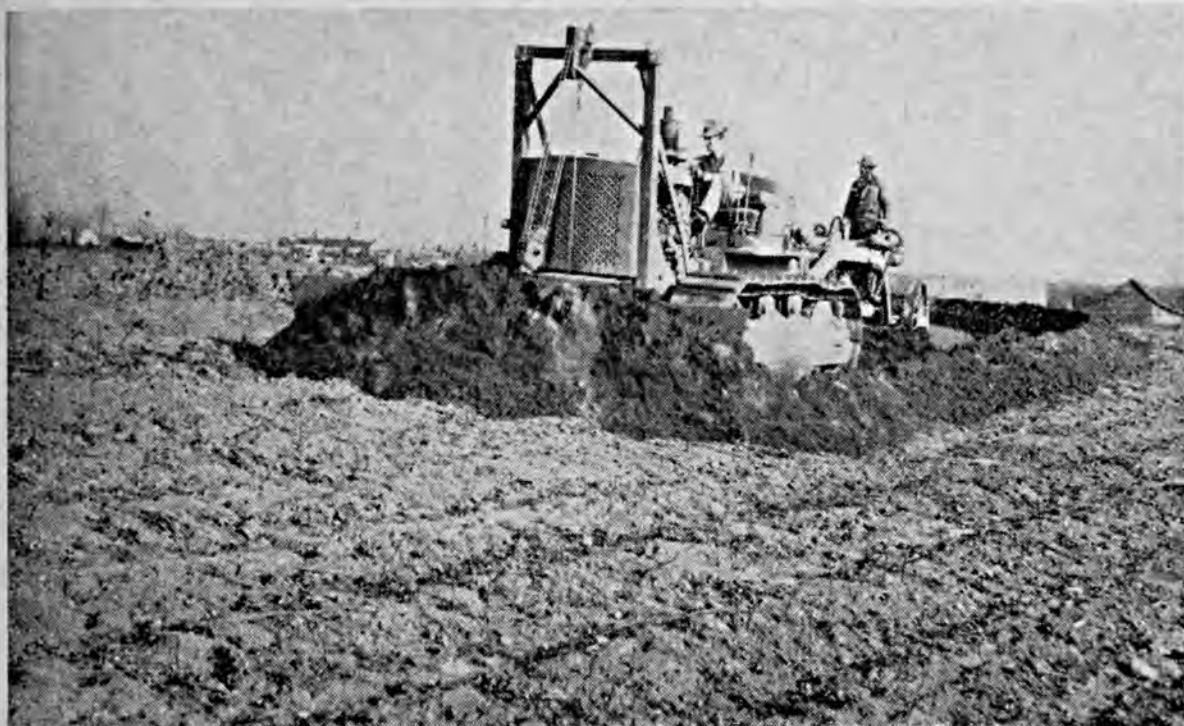
Fig. 2. Heavy equipment, privately owned, furnishes power to build terraces, dig the canals, make farm ponds, and convert handicapped or idle land into useful, working acres.
