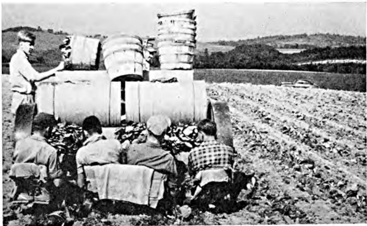
Fig. 4. This cabbage transplanter places the fertilizer in bands and applies starter solution.
