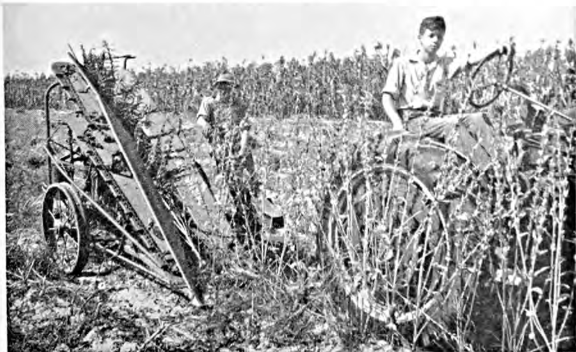
Fig. 4. A tractor and corn binder were used at Florence, South Carolina, to harvest an acre of sesame in 1\frac{1}{4} hours, requiring only 2\frac{1}{2} man-hours. Hand-harvesting operations take approximately 30 man-hours per acre.
