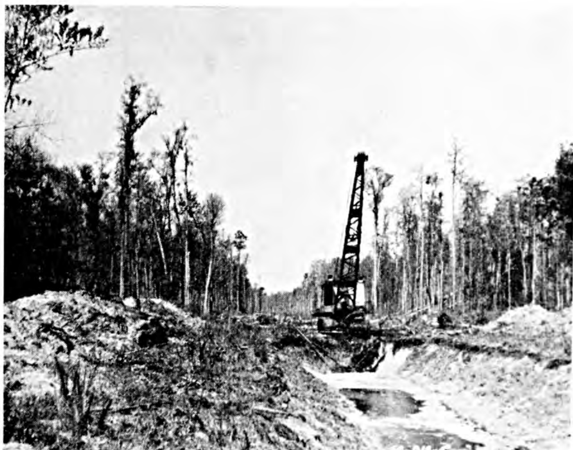
Above: Dragline excavating a main canal on the Cypress Woods plantation in Jasper County.
