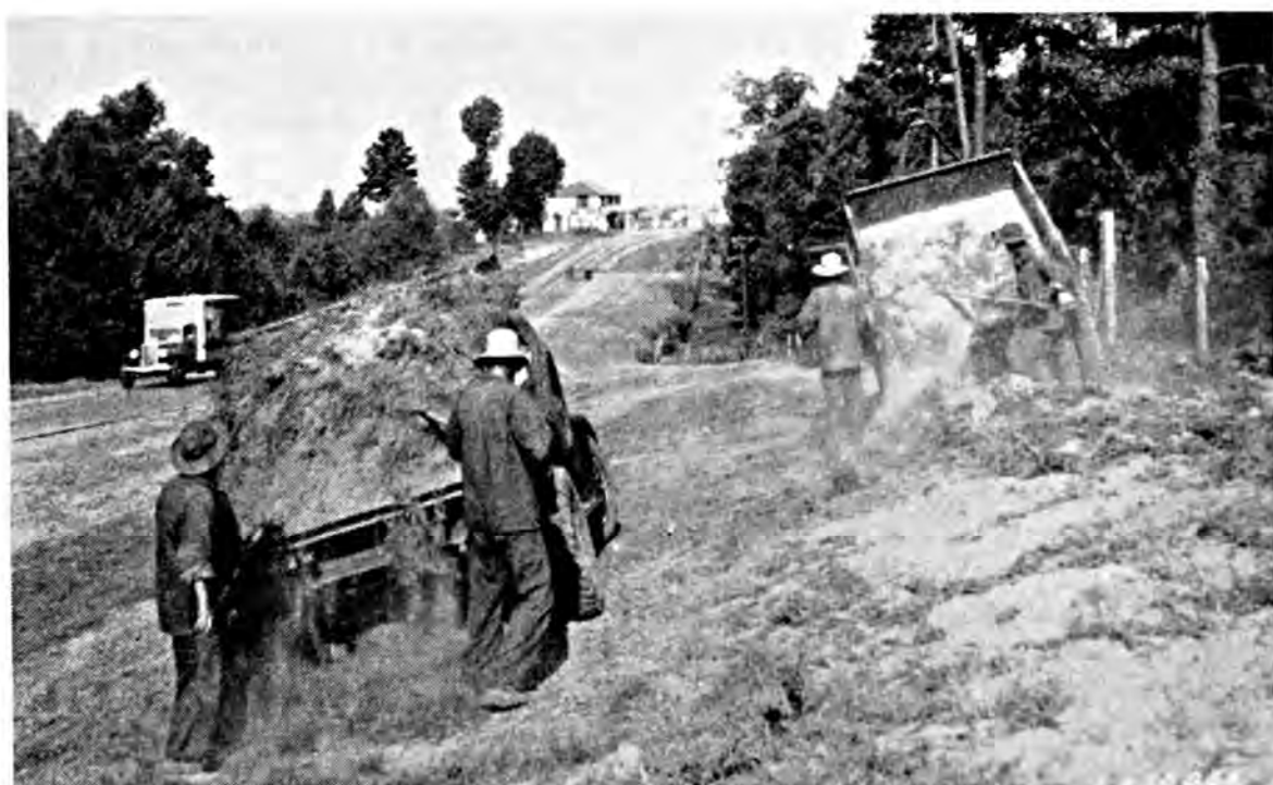
Fig. 2. This highway crew is sodding Bermuda-grass for erosion control near Minden, Louisiana.
