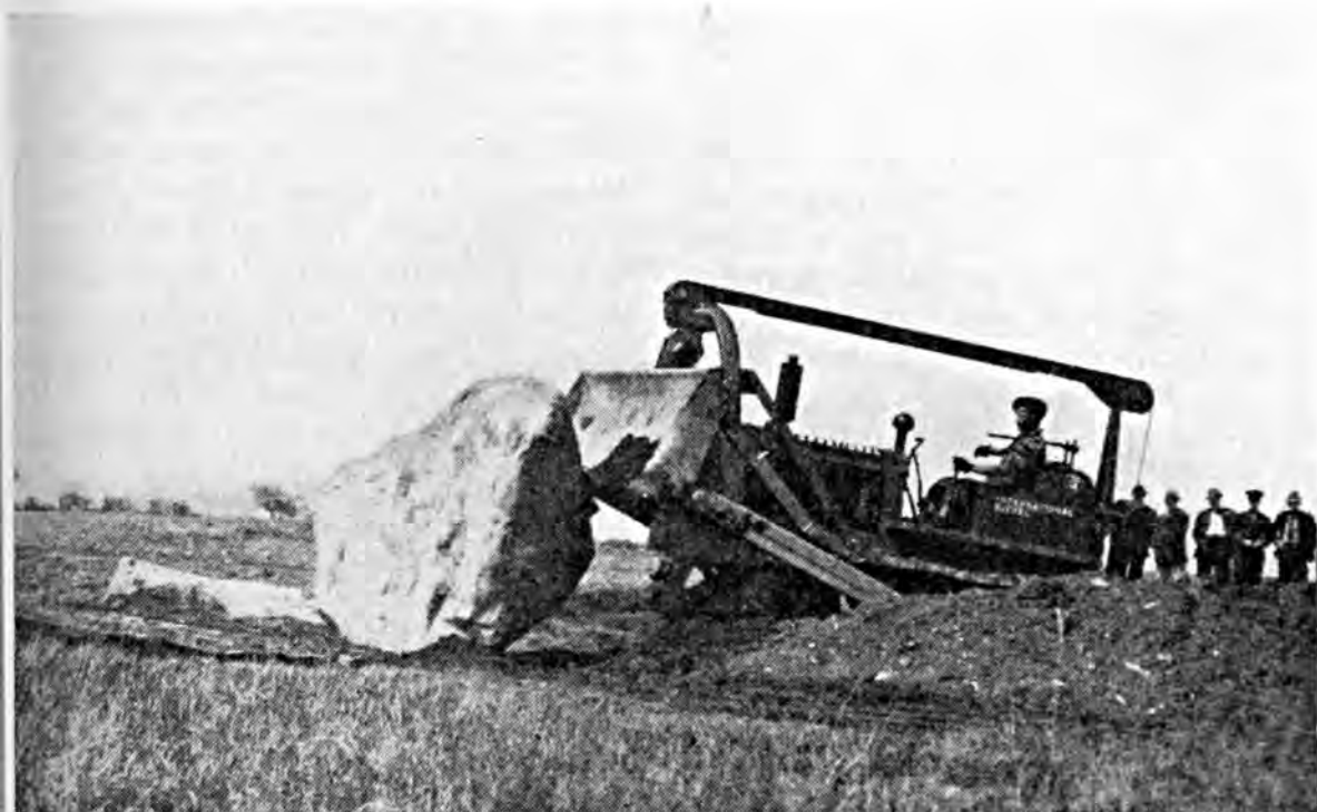
Fig. 1. With a push here and a shove there, this bulldozer operator rolls a huge boulder onto a giant, steel stoneboat.
