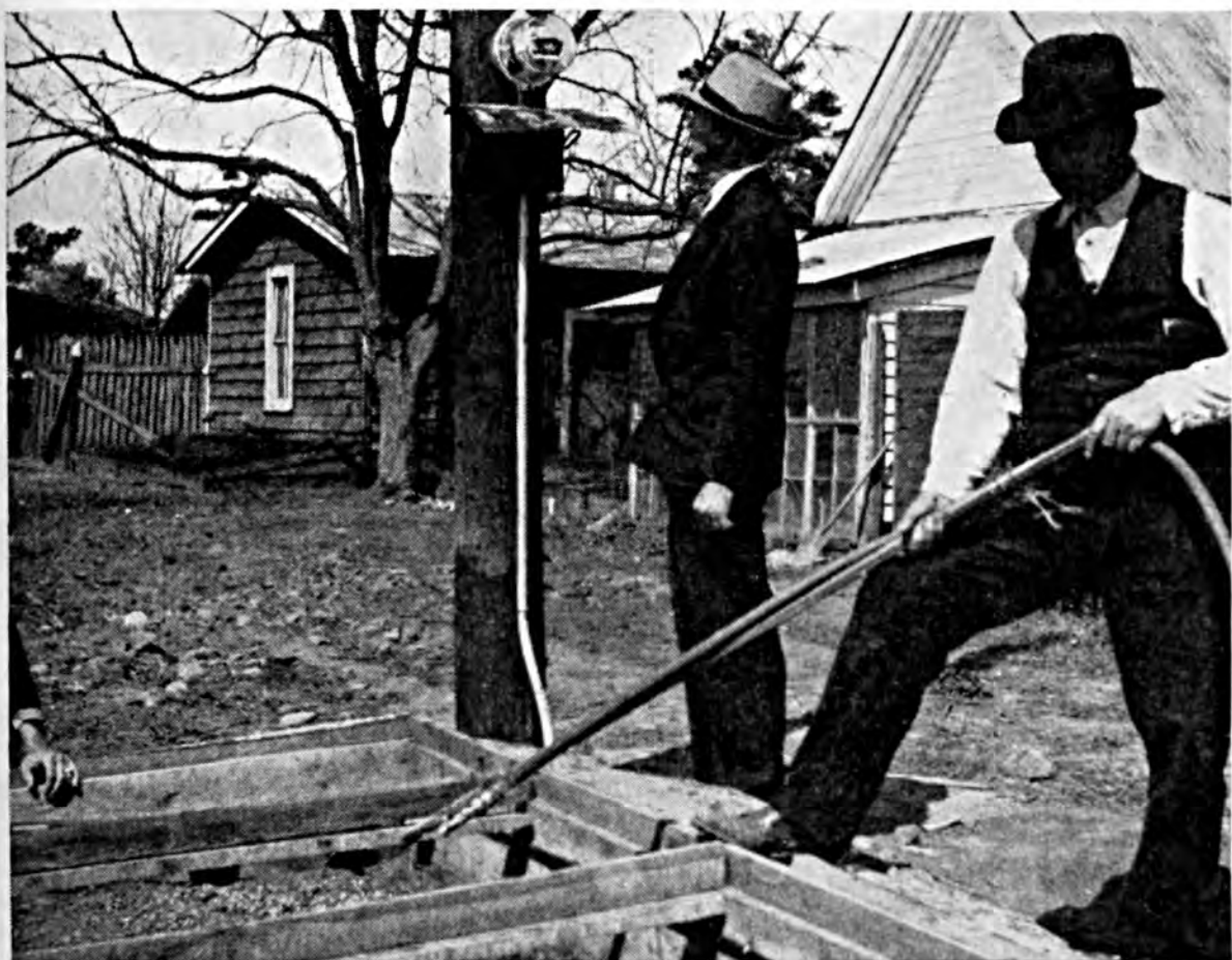
Above: Here is an electrically heated hot-bed for sweet potato plants used by Walton farmers.
