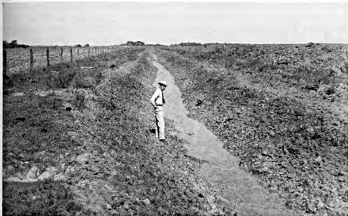
Fig. 3. Bob Harling, Soil Conservation Service technician assigned in the Trinity Bay Soil Conservation District, inspects a drainage ditch built on the G. R. Canada ranch. Engineers from Mr. Harling's office helped Mr. Canada lay out the ditch lines as part of the soil conservation program being installed on the ranch.
