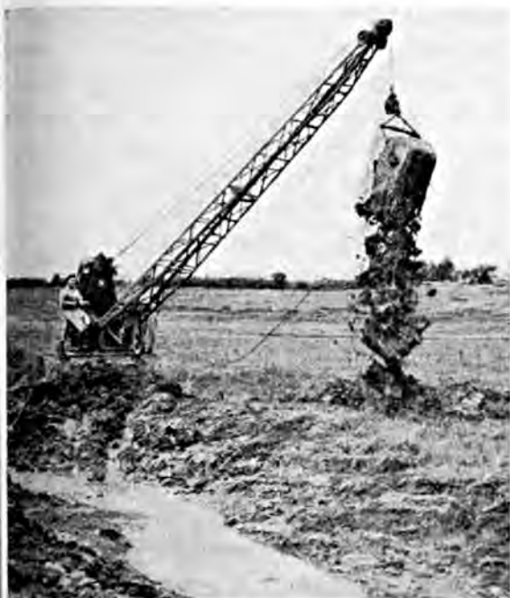
Fig. 3. A dragline does the "dirty" work in large drainage ditch construction.
