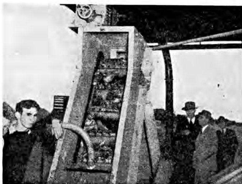
Showing washer-elevator at Perry, Georgia. The potatoes are washed, crushed, dried, and sacked.
