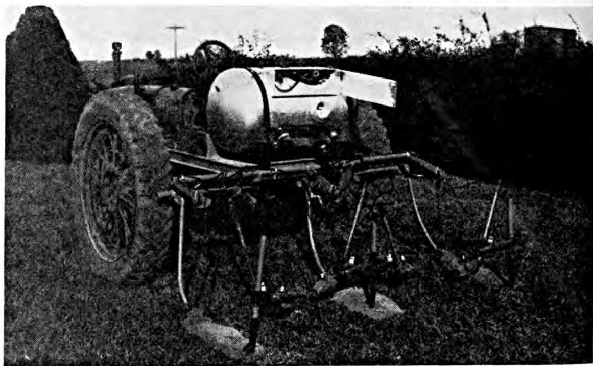
Fig. 6. An experimental two-row flame cultivator for use of compressed gas.
