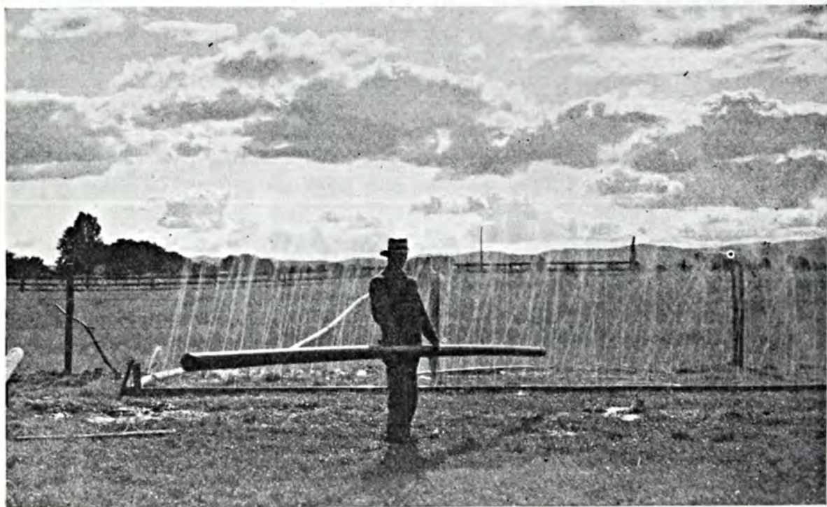
Perforated pipe operating at 15 pounds pressure.
