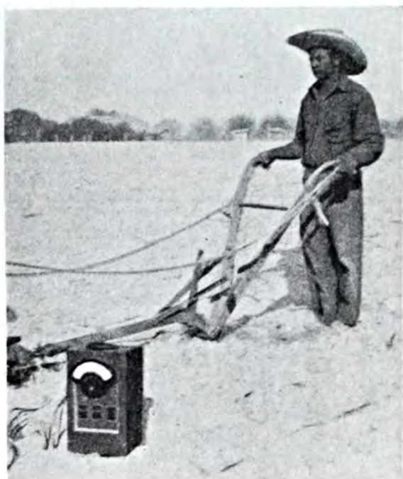
Fig. 11. (Right) Dynamometer on plow for opening furrows—Method No. 6.
