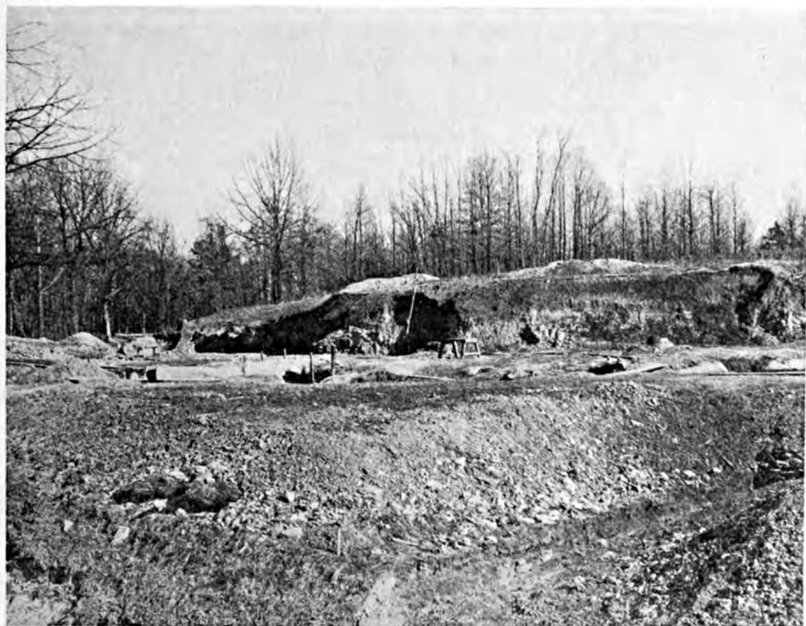
Below: Limestone rock quarry being stripped in Hopkins County, Kentucky.
