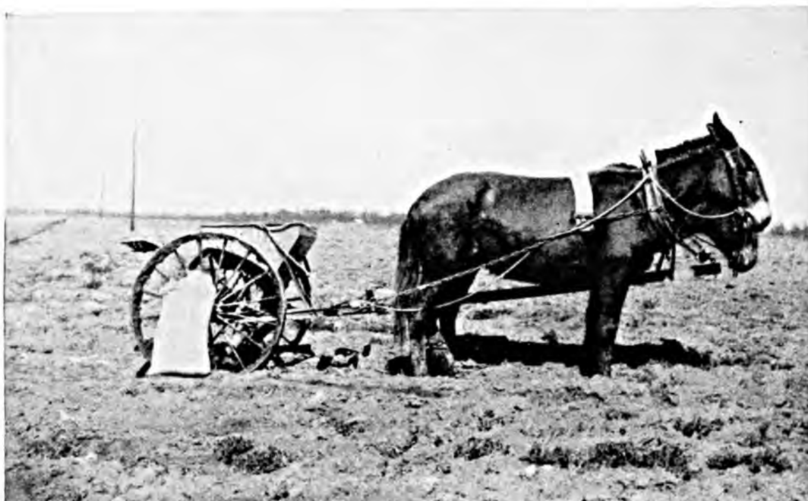
This two-row distributor in common use in Mississippi, more especially in the delta, is adapted for applying fertilizer in drill before bedding land. Applications should be made 10 days to 2 weeks before planting.
