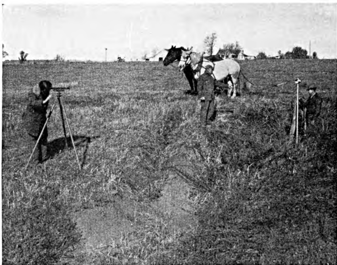
Above: Planning outlet for contour stripping system in Illinois. Waterway will be bladed in and seeded, and sod flume will be constructed.
