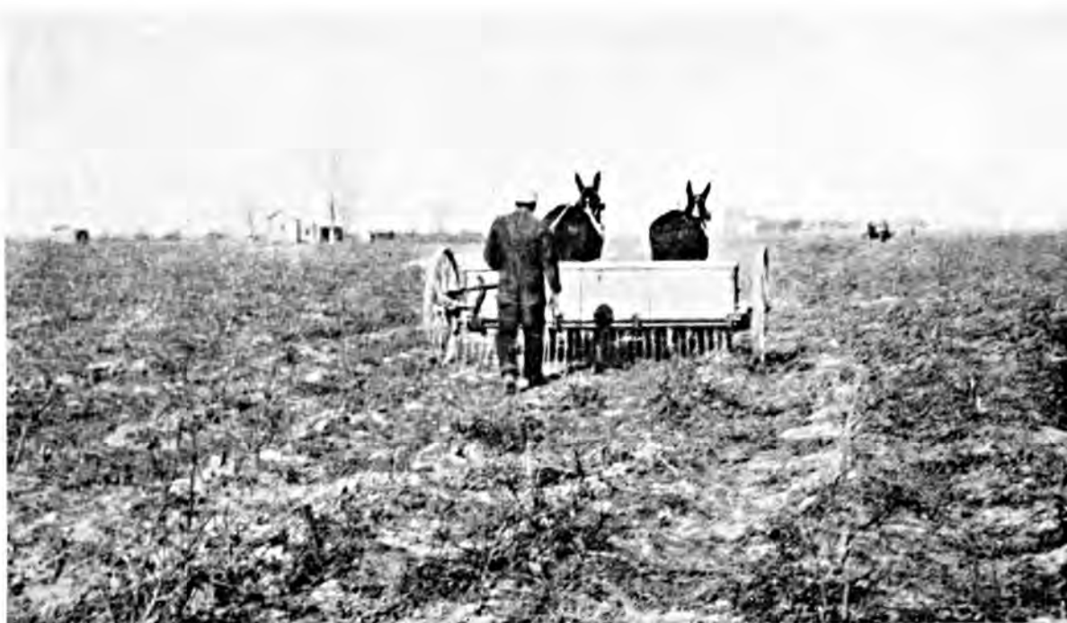
The broadasting type of fertilizer distributor in common use in Mississippi, especially the delta, is well adapted for pastures, hay crops, and small grains.
