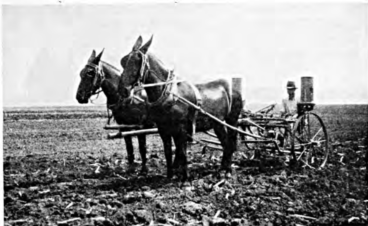
This distributor attachment for cultivators is commonly used in the Mississippi delta for side-dressing.
