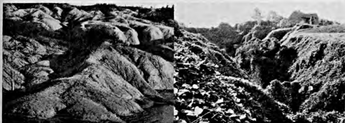
Left: On this land CCC workers have built brush dams for the control of gullies. Eventually trees and vegetation will help nature rebuild. Right: Kudzu or "porch vine" used to stabilize gullies and on badly eroded fields also provides excellent forage. Since it is a legume it enriches soils that are very erodible.
