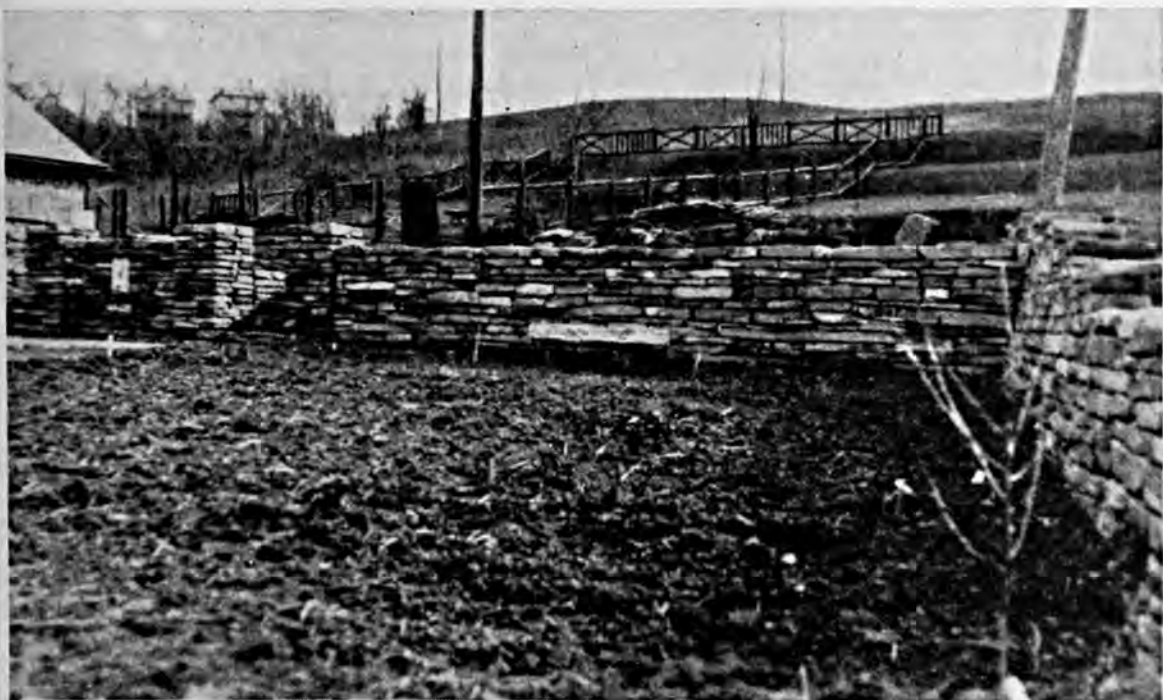
This yard after grading has dry stone walls to maintain grade differences.
