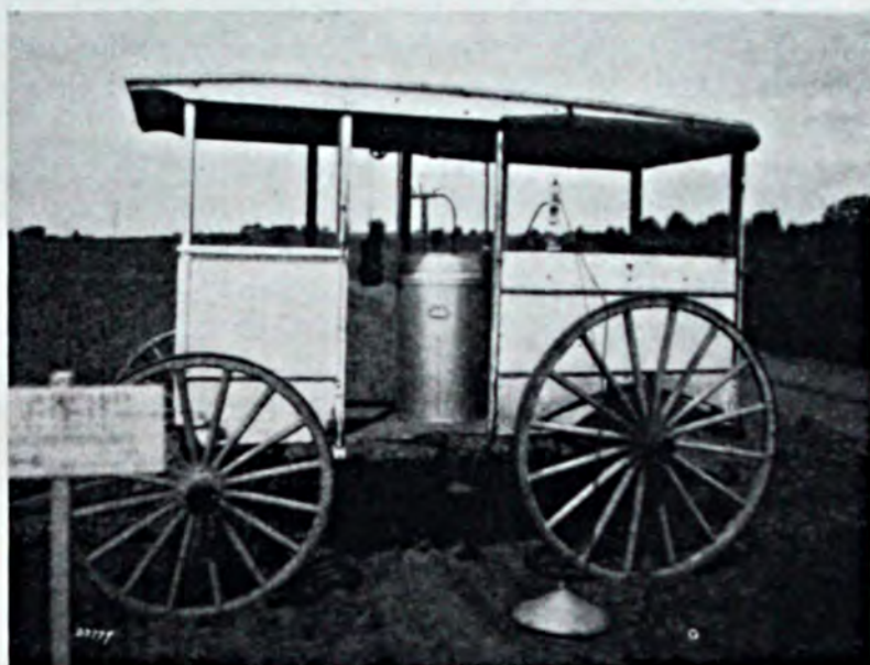
A milk wagon was remodeled for the equipment with which Professor Smith took the respiration of the soil. With this outfit he has found that the productivity of the soil is directly related to the amount of carbon dioxide it produces.
