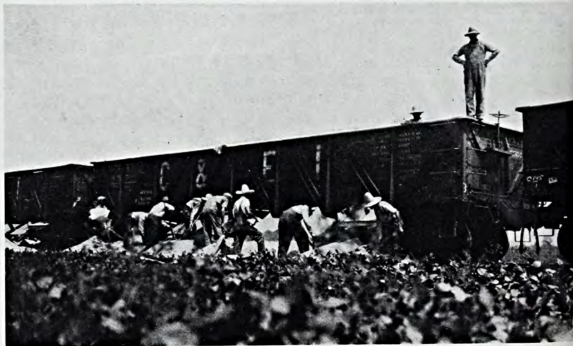
This trainload of limestone is being unloaded on right-of-way from side-dump cars.
