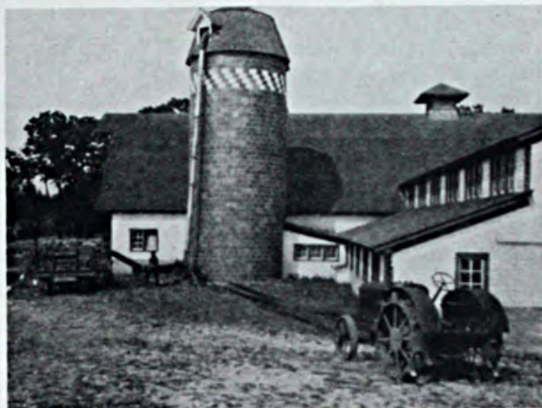
With equipment like this, a silo can be filled at the rate of 20 tons per hour.
