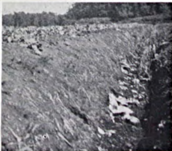
Below: The same ditch a few weeks after spraying with calcium chlorate. Note the clean and neat appearance.
