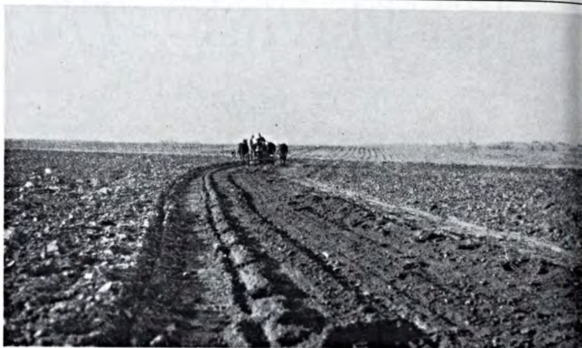
Here a terrace is being constructed to carry water off from the adjoining fields.
