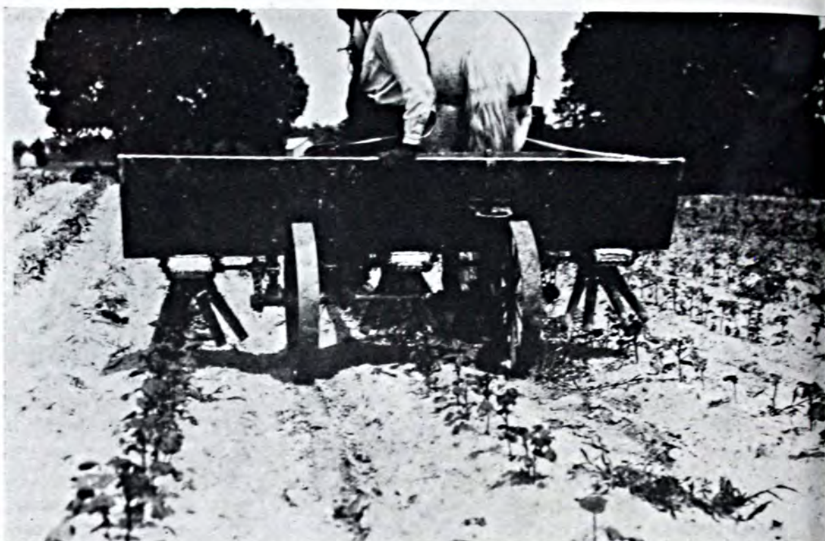
Mr. W. T. Moss of Youngsville, N. C. rigged up a new kind of distributor for putting out his potash top-dresser.
