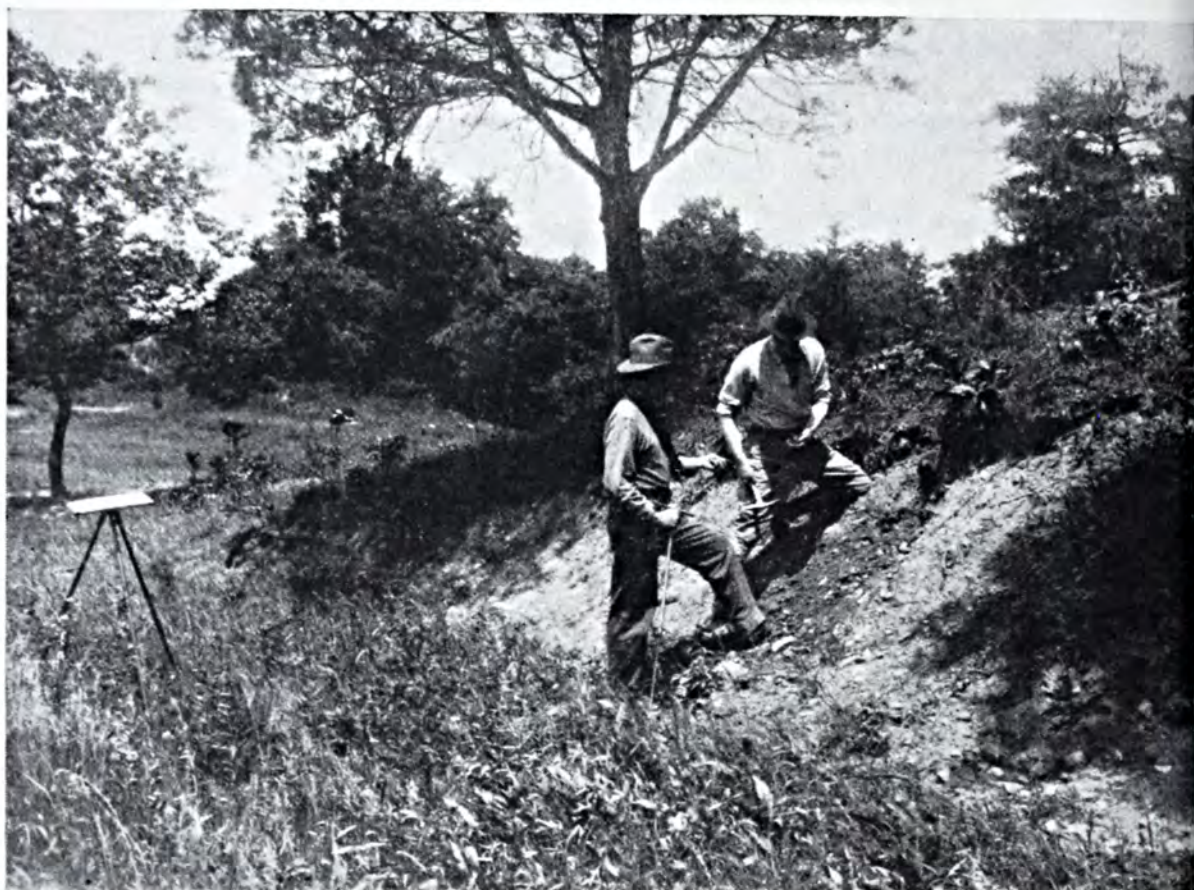
New road cuts and ditches are always welcomed by the soil survey man. From these he can obtain the best possible idea of the surface soil, subsurface, and subsoil, the underlying strata, and also the color, texture, and structure of these.
