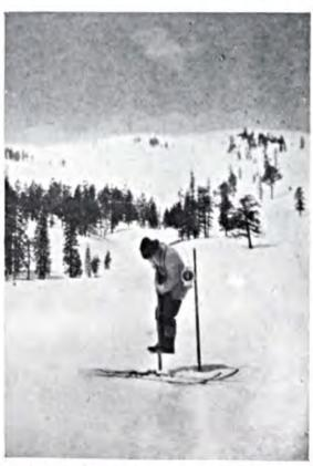
Driving the sampler in deep snow at Ward creek (elevation 7,000 feet) at the eastern crest of the Sierra Nevadas.
