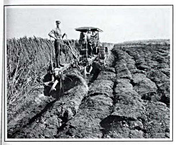
Breaking Hollandale muck soil with a 10-ton tractor hooked to two 26-inch plows that turn a furrow 10 inches deep and bury the heavy growth of wild rice and other swamp plants.
