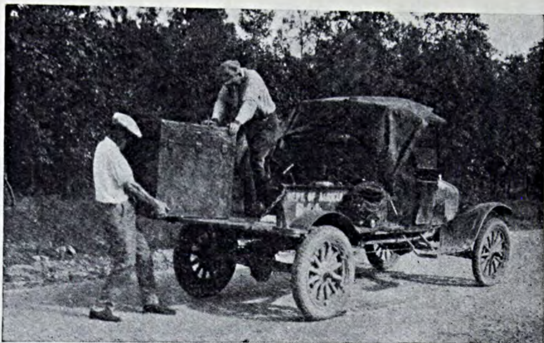
The U. S. motion picture truck carries portable projector, generator, batteries, electric lights, power cable and repair parts. The outfit shows clear, bright, first-class pictures.
