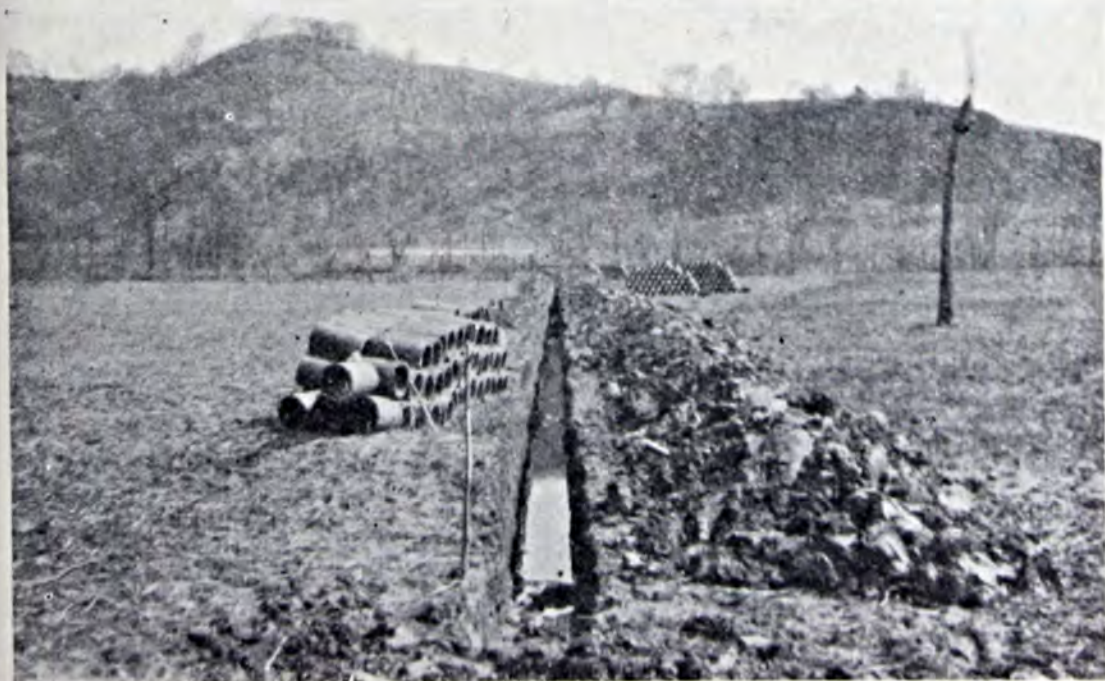
Beginning work on the new system of drainage on the Robinson farm.
